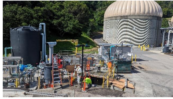
4/16/2024: Construction of widened hatch
