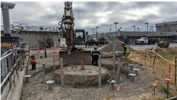
7/10/2023: Helical Piles for tank foundation
