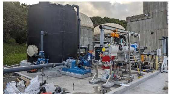
1/3/2024: Installation of pipe/equipment
