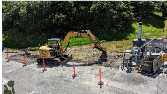
04/25/2023: Site prep for construction
