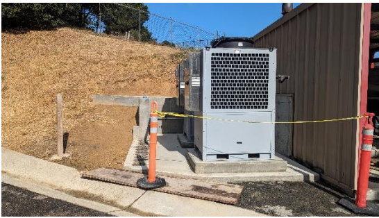
9/14/2023: Installation of chillers
