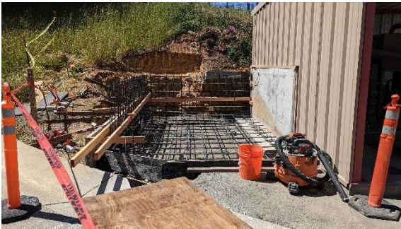
5/11/2023: Biogas Foundation Construction
