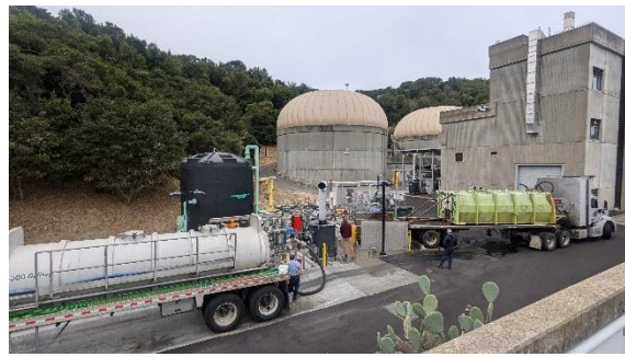
9/20/2024: Use of new tank & widened hatch
