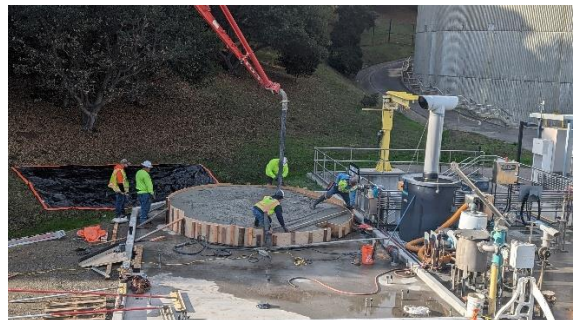
11/21/2023: Forming concrete pad for tank
