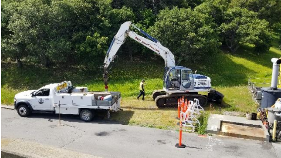
04/21/2023: Geotechnical test pile
