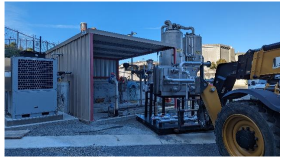
11/27/2023: Installation of heat exchanger
