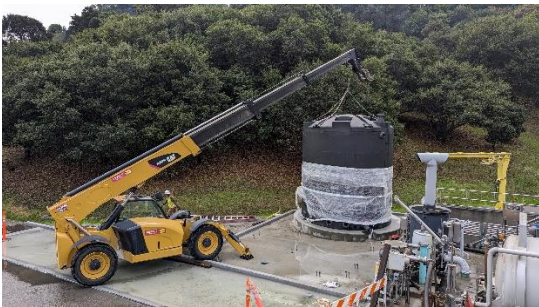
11/29/2023: Installation of new tank
