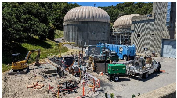
5/15/2023: Excavation for tank/piping
